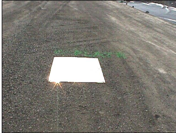
Figure 1: Copper plate under 21-B material in section B.
