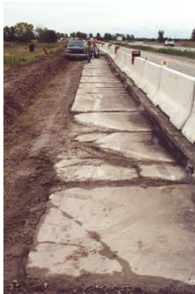
Figure 4. Typical concrete road base condition in eastern PMS sections (near Tilbury).
