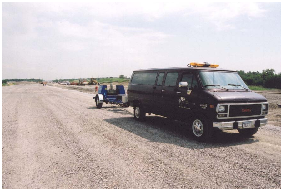
Figure 1. FWD Testing on Top of the Granular Base Layer.
