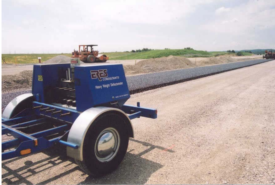
Figure 2. Close-Up of FWD Testing the Top of the Granular Base.
